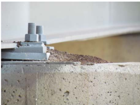
Photo 5: Guano deposit on pier, obscuring structural features.
