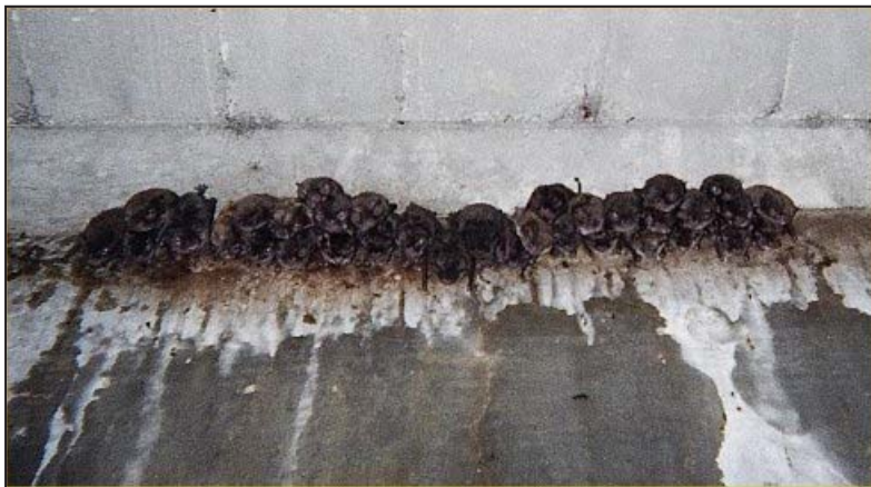
Photo 11: Bats Roosting & Associated Staining
