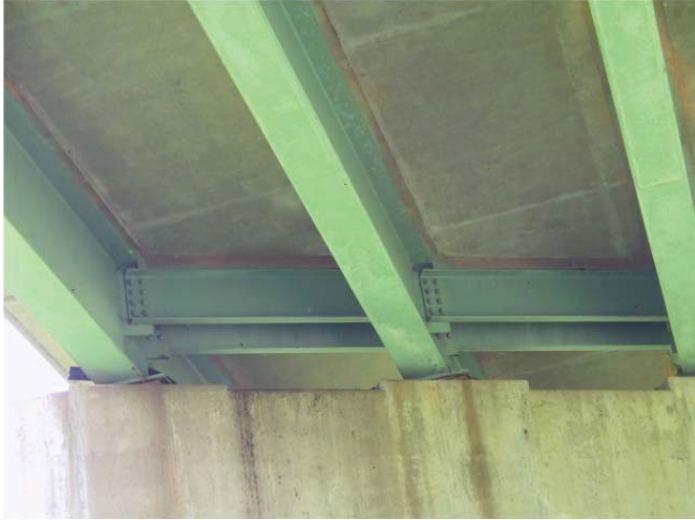
Photo 10: Guano staining on side of pier
