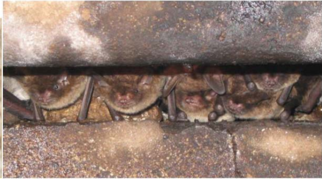
Photo 2: Visible bats within an expansion joint
