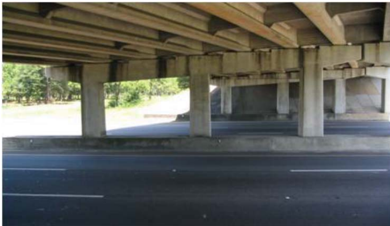
Photo 9: Staining on sides of pier caps
