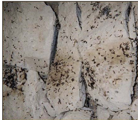
Photo 6: Bat Guano on Riprap
